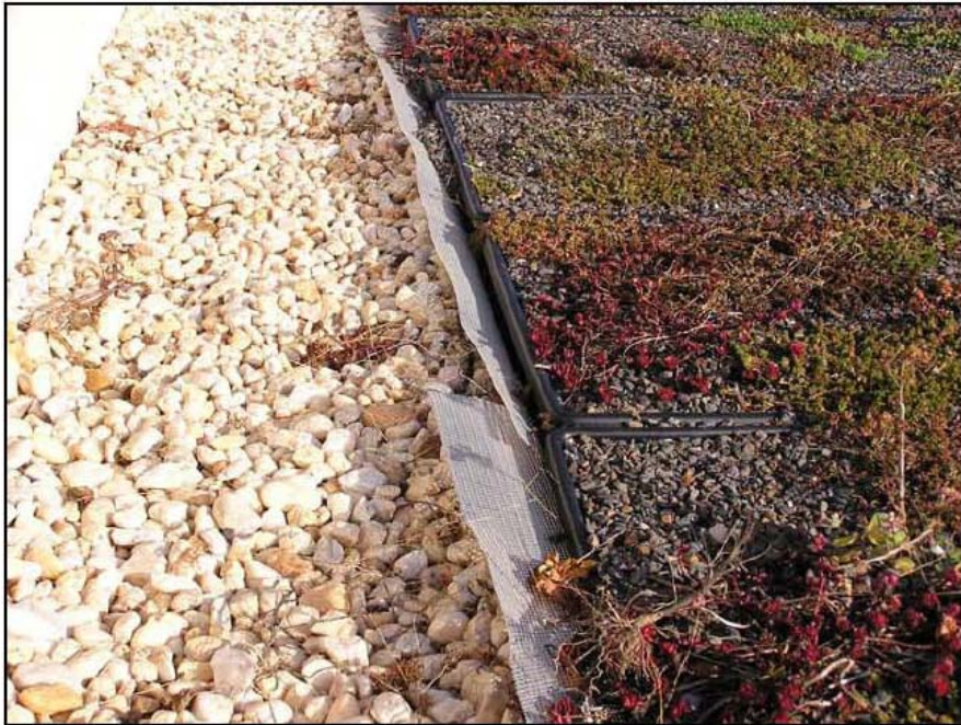
Aluminum edging falling apart and protection fabric not UV stable.
