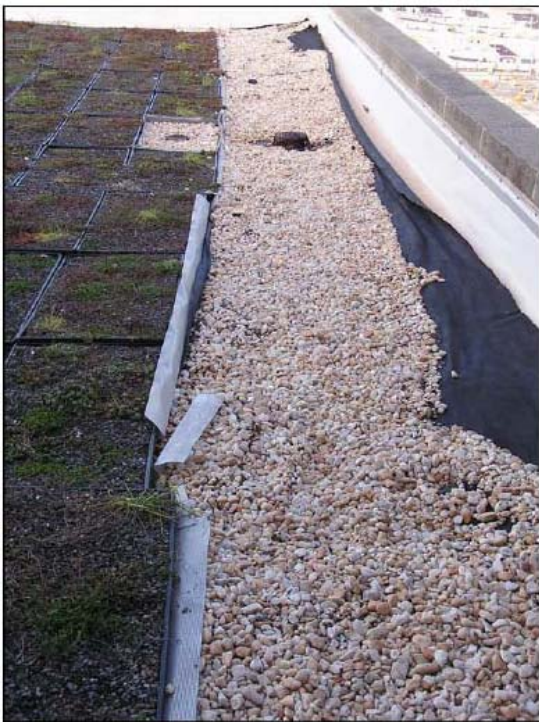
Aluminum edging falling apart and protection fabric not UV stable.
