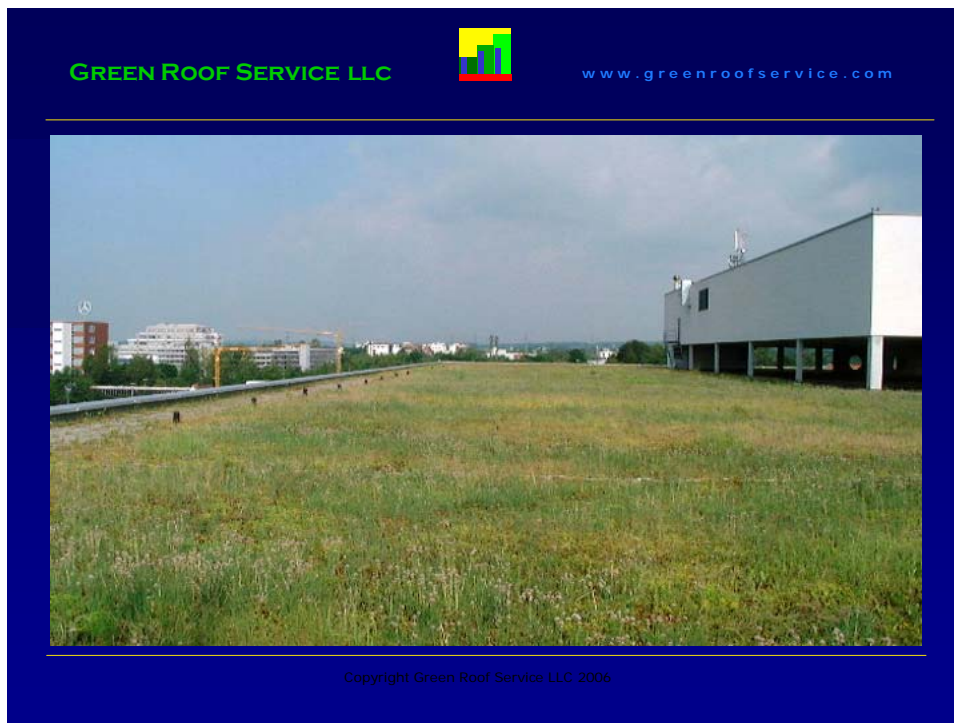
Photo 5: Typical German eco-roof in single course construction
