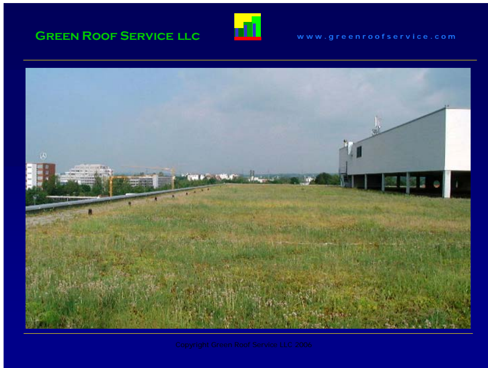
Photo 5: Typical German eco-roof in single course construction
