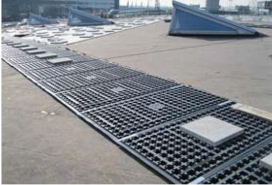
Roof penetration: Solar Base SB 200 elements are used for the subsequent installation of the solar modules and are held in place by the ballast provided by the roof substrate.
