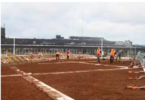
The roof substrate provides the required ballast for the Solar Base
