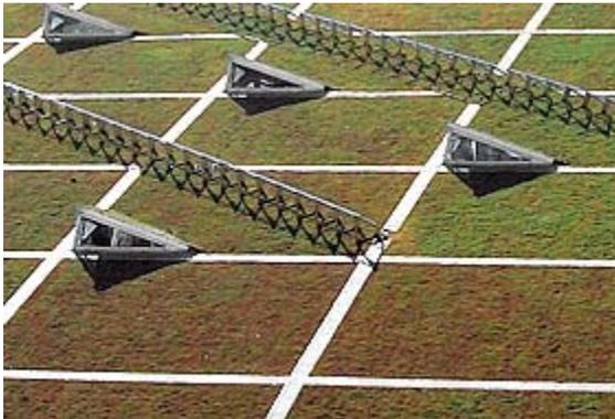
The geometric arrangement of the rows of solar modules and the pathways between the skylights resulted from the load-bearing capacity of the roof.
