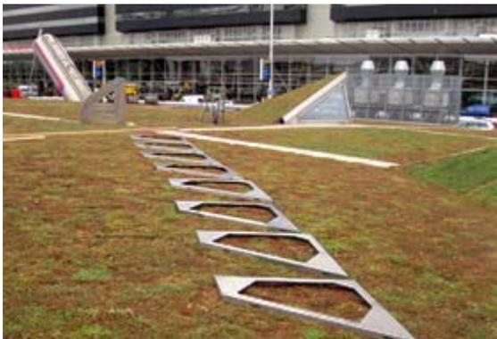
The Solar Base Frames can be set up either before or after the plant layer has been installed. Things were very flexible in this respect at Schiphol Airport.
