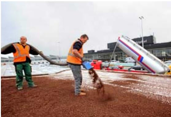
Using silo vehicles, the system substrate "Sedum Carpet" is blown onto the roof where it is immediately distributed.
