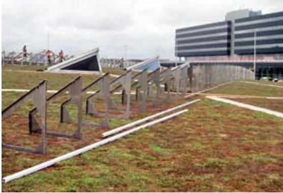
The existing roof pitch was not a problem when installing the rows of solar modules.
