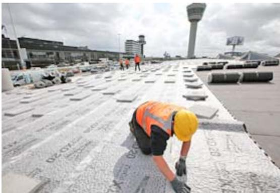
With anti-slip mat: ZinCo supplied the laminated drainage sheet Fixodrain® XD 20 with an additional rubber protection layer on the underside specially for Schiphol.
