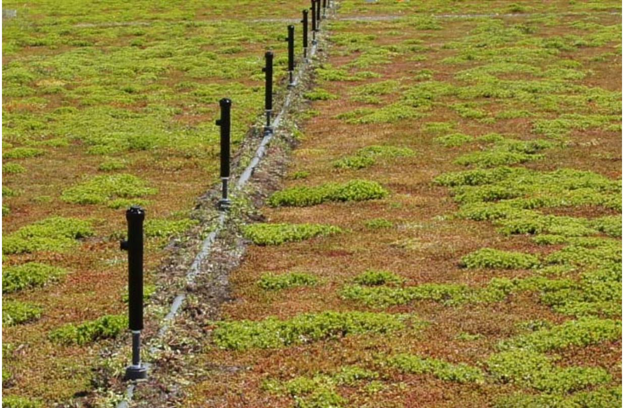
A permanent irrigated extensive Green Roof with sprinkles – most inefficient and most plants destructive solution. Photo: Jörg Breuning
